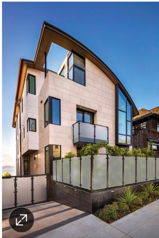
Construction of the limestone house took almost four years, said developer Bill Campbell of Marble Management. PHOTO: JACOB ELLIOT PHOTOGRAPHY
